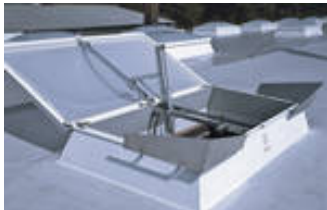
Natural smoke extraction
