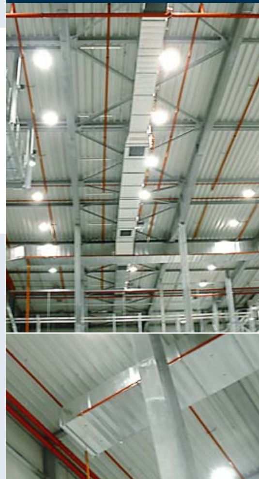
Duct system instead of roof openings
