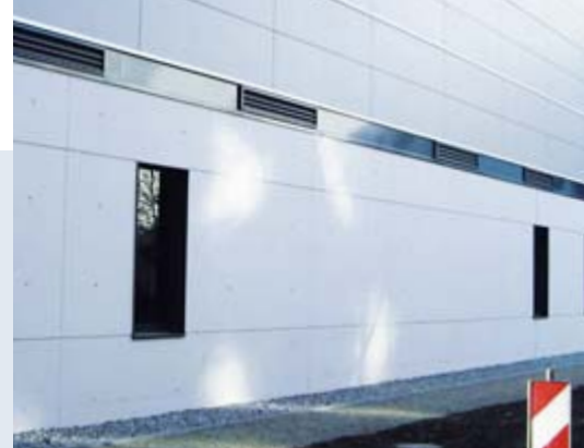
Front view of car park with SHE ventilation components
